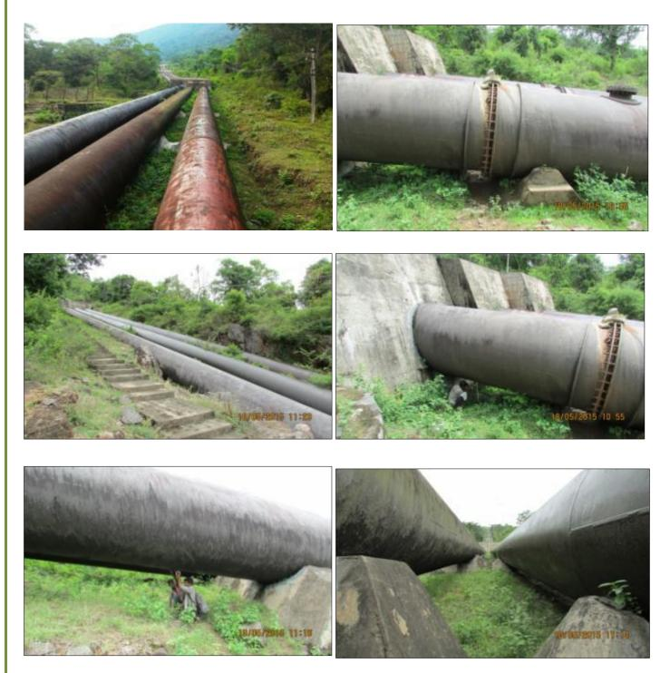
Top left: A view of Parali penstock pipeline, Top right: Water leakage in the pipeline joint, Middle left: Shows suitable place making ramp/overpass to facilitate animal movement, Middle right & Bottom left: WTI team measuring gap between pipe and ground, Bottom right: Close up view of alignment of parali pipeline.
